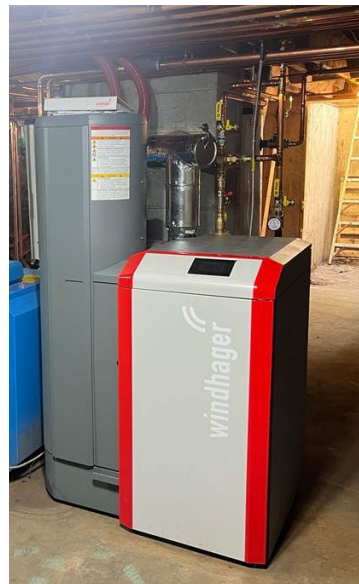
Figure 7. Old coal/wood combo boiler (left), and new pellet boiler (right) in Groton.
