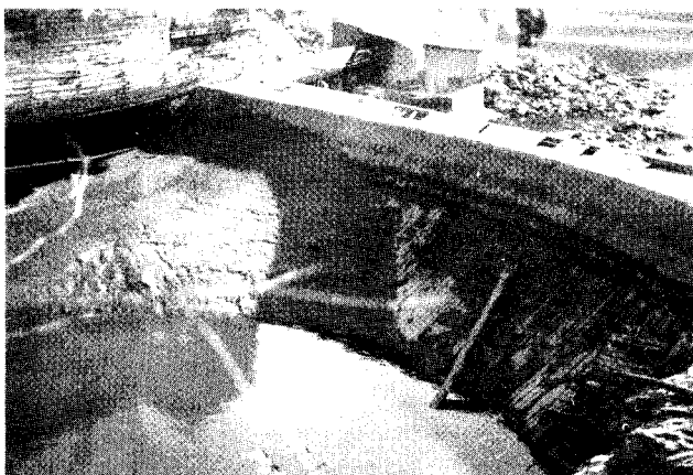
Figure 3.3 Impoundment Siltation. Drawdown behind the dam has revealed a quantity of Winooski River silt.
