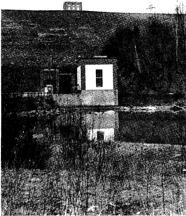
Figure 2.6 A Modern (1950's) Powerhouse. The power facility is an addition to a flood control dam built in the 1930's.
