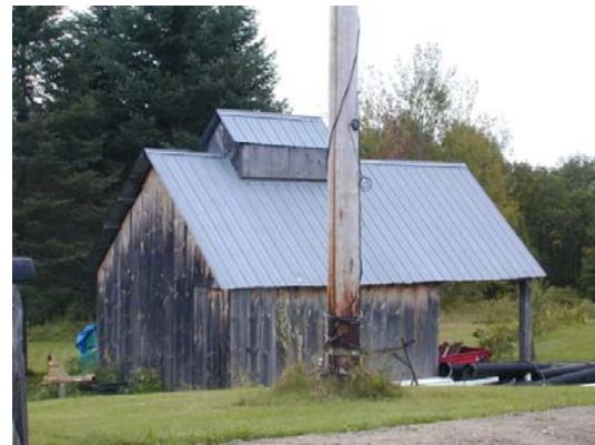
An equipment shed near the turbine houses inverter and transformer
