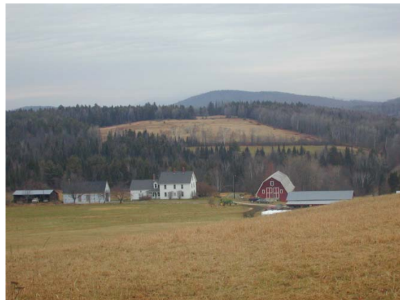
A buried conduit connects turbine generator and wind equipment (behind photographer) to the basement of the white house at center
