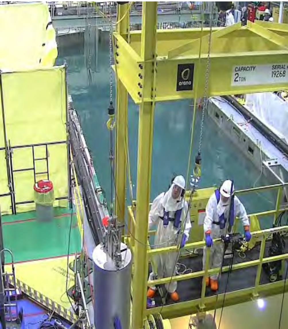
Installing collection barrel in the Filter System
