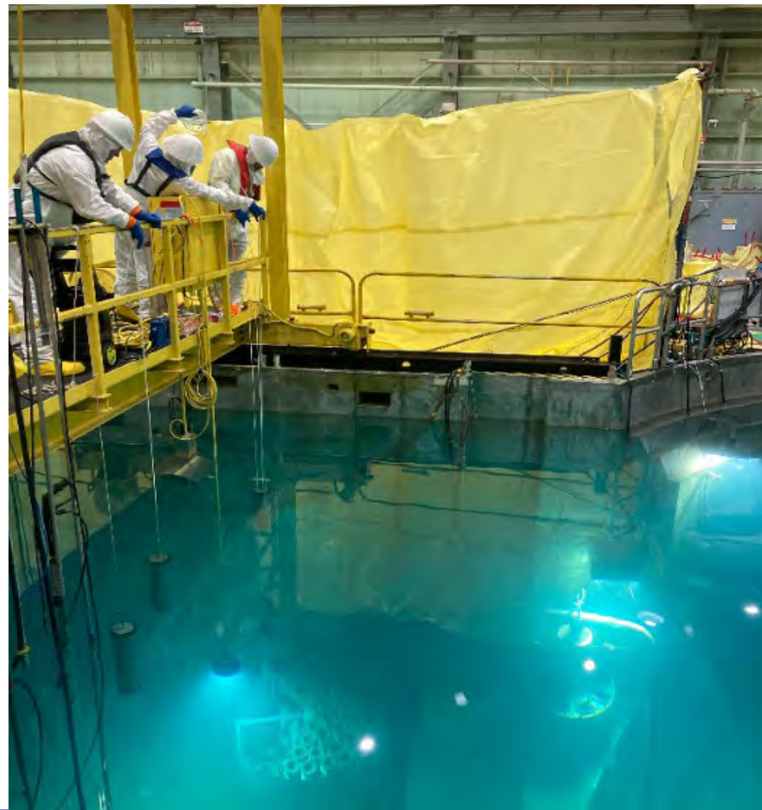
Installing collection barrel in the Filter System
