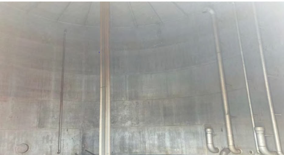
Set up for tank interior piping removal
