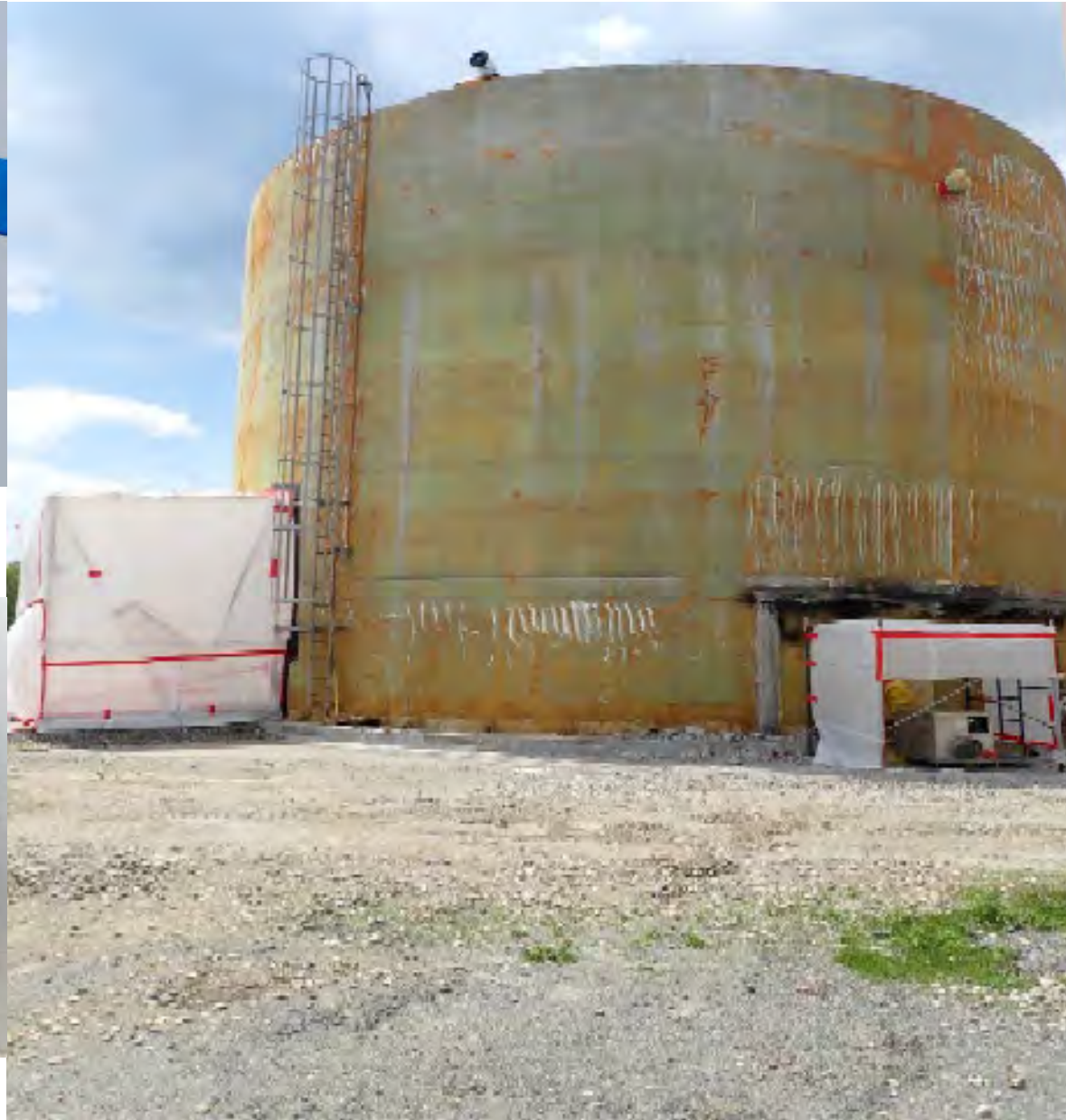
Set up for tank interior piping removal
