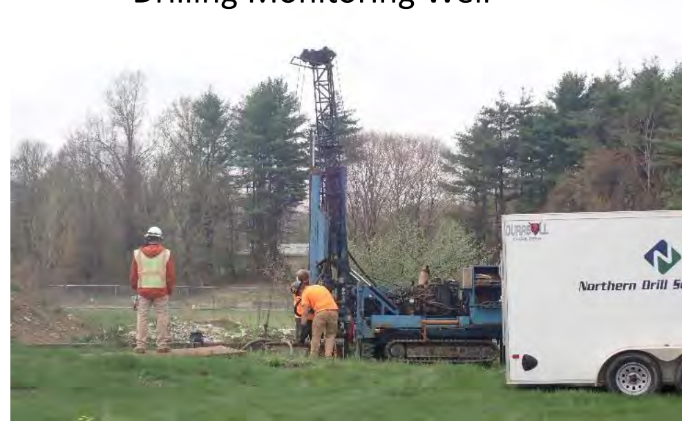
Drilling Monitoring Well
