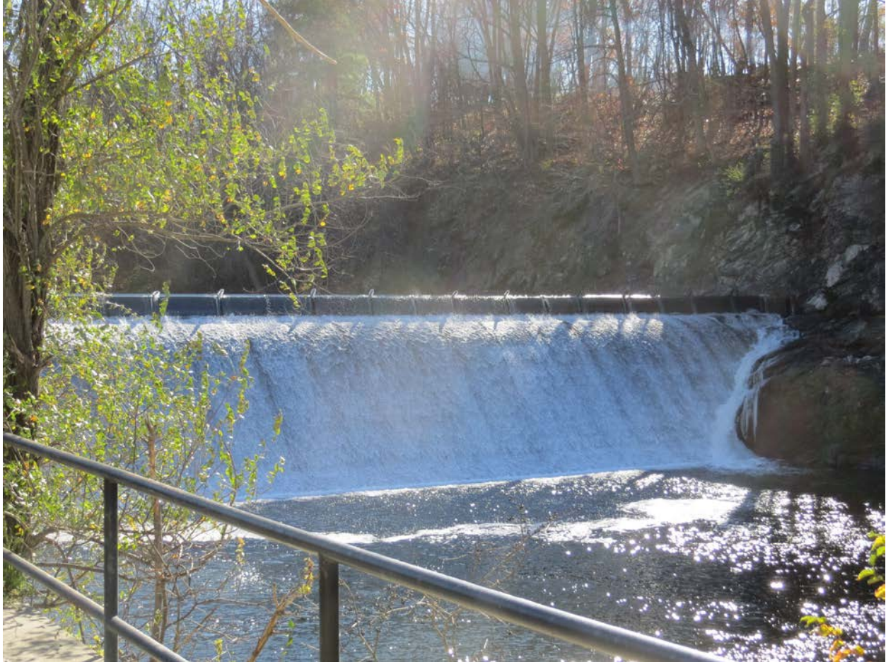
Above: 500 kW hydropower project in North Pownal, redeveloped by Hoosic River Hydro in 2017. Credit: Jim Therrien, New England Newspapers
