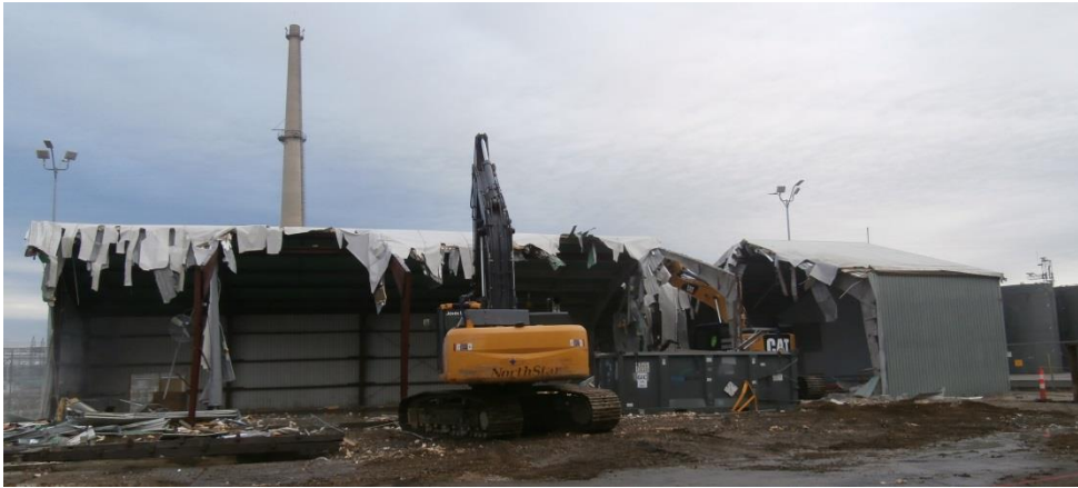
North Warehouse Demolition
