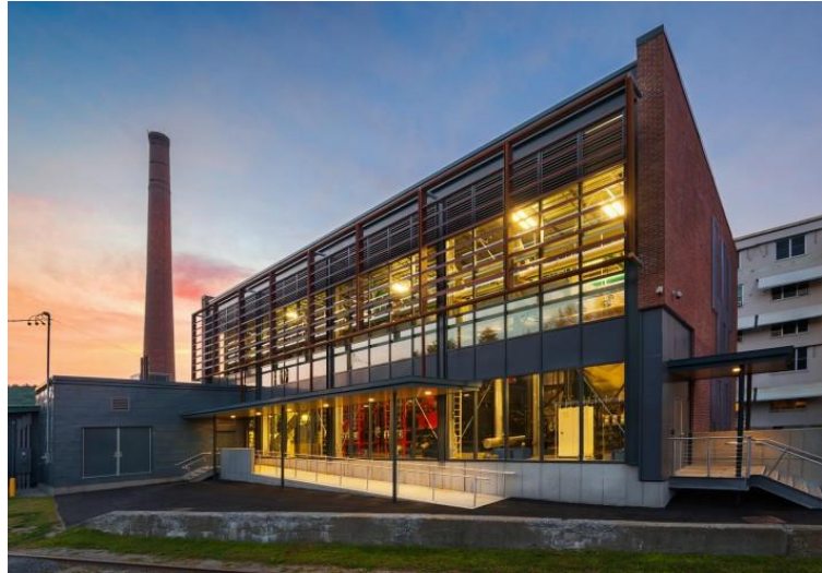
Montpelier District Heating Plant Photo Credit: Gary Hall
