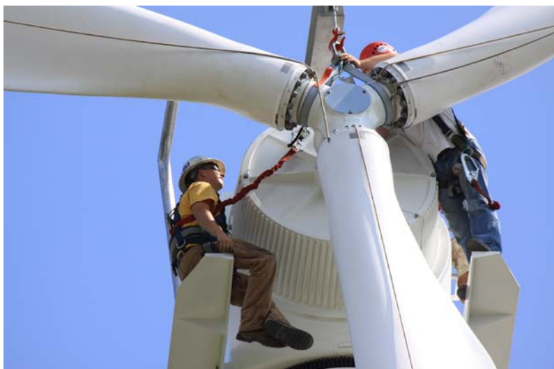
Installing a Northwind 100 kW turbine in Barre, Vermont. Photo by Northern Power Systems, Inc.
