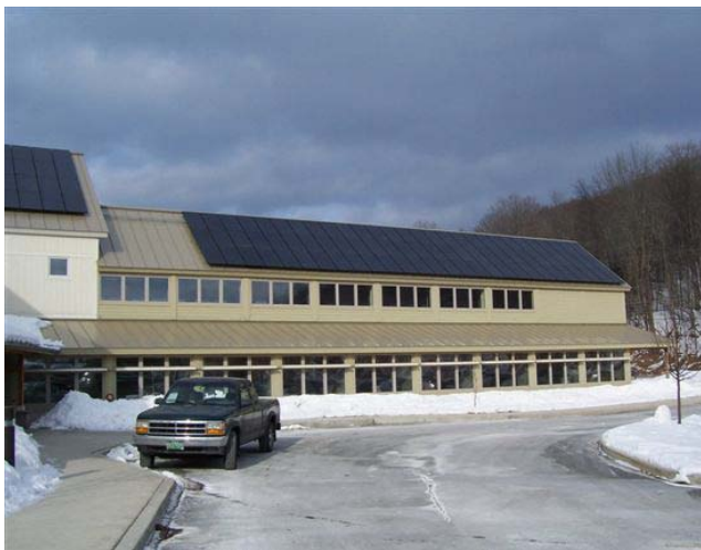
38 kW Solar PV array installed at the Health Care & Rehabilitation Services of Southeastern Vermont, Inc. with a CEDF state grant. (Photo provided by Health Care & Rehabilitation Services of Southeastern Vermont, Inc.)
