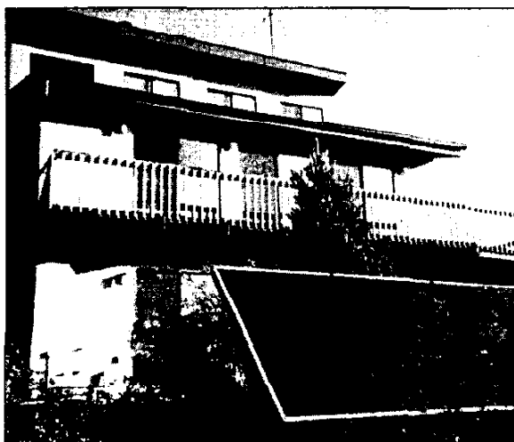
Nestled into the hills 18 miles north of Prescott is this PV and passive solar home. Photo by Bob Hammond.
