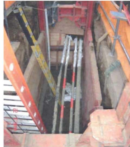
AOG Pipe Tunnel Excavation
