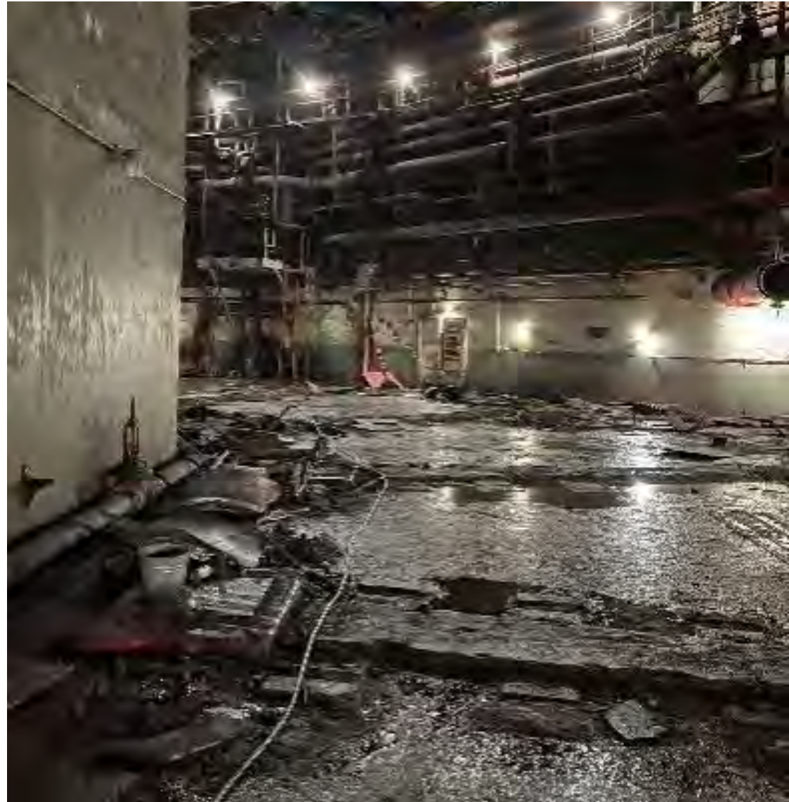
TORUS Demo & Removal Complete
