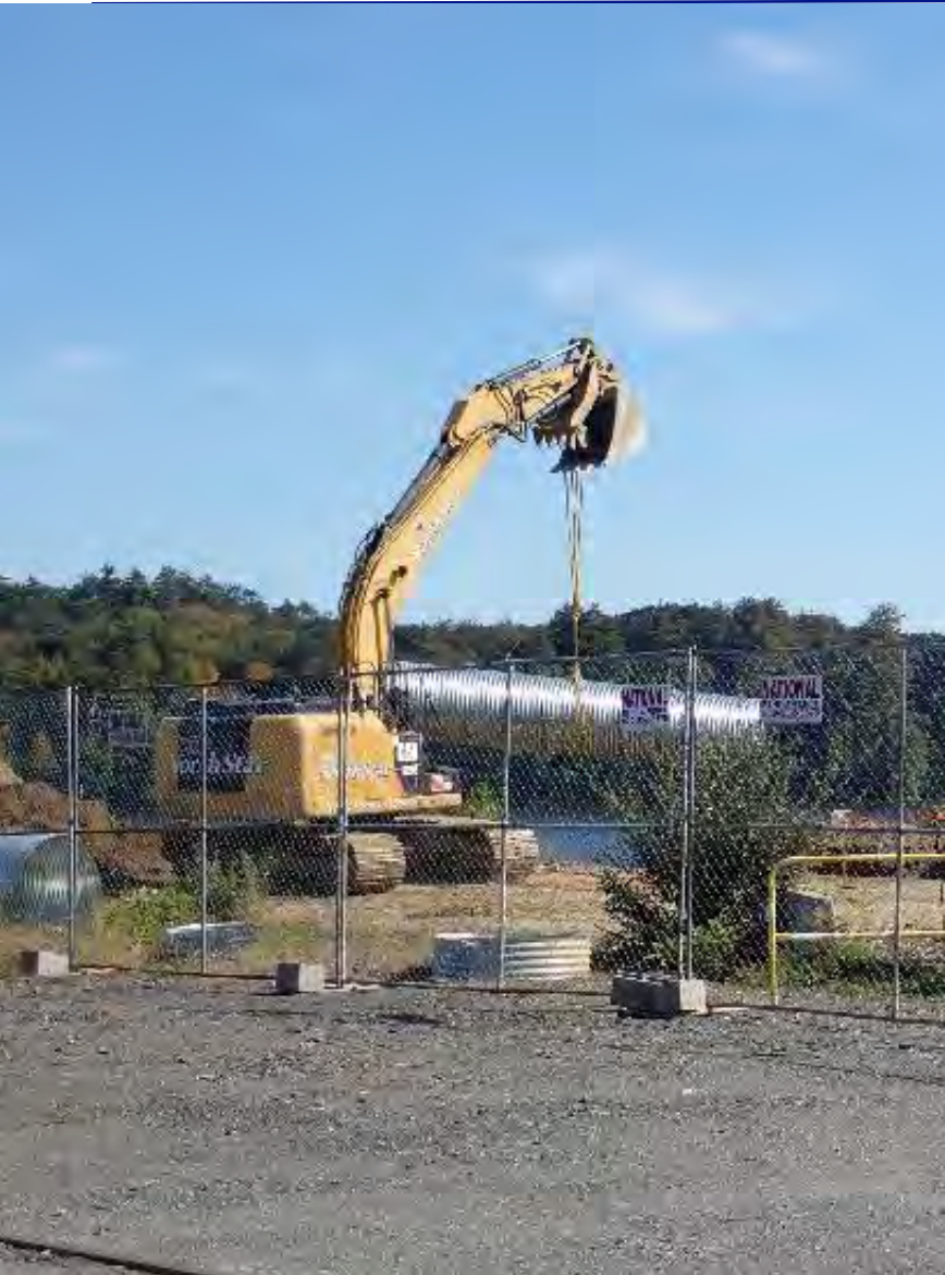
Rerouting Stormwater Drain Line at North end of Discharge Structure
