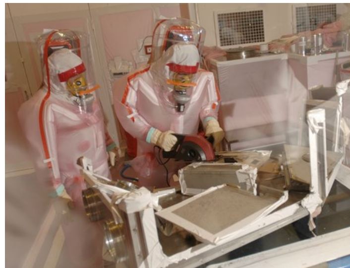
Dismantling mixed oxide production facility
