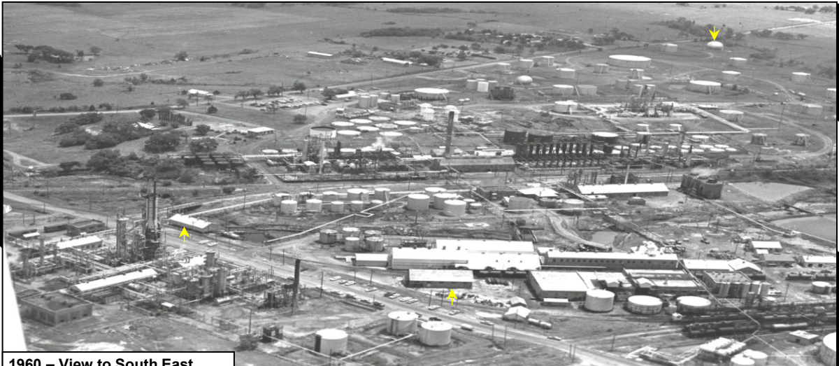
1960 – View to South East
