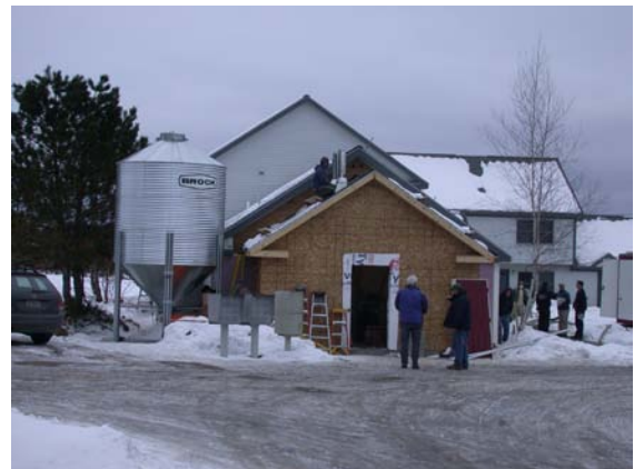
Photo supplied by Housing Vermont
