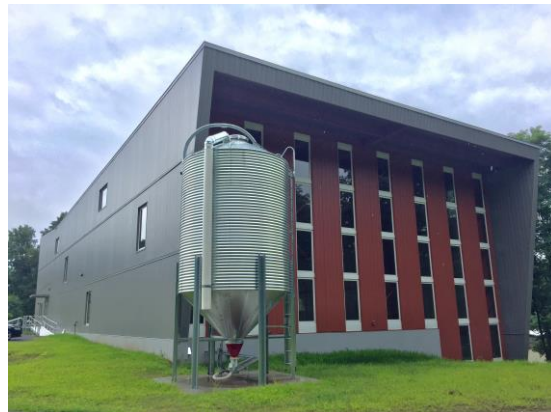
New England Center for Circus Arts storage silo for advanced modern wood pellet heating system in Brattleboro
